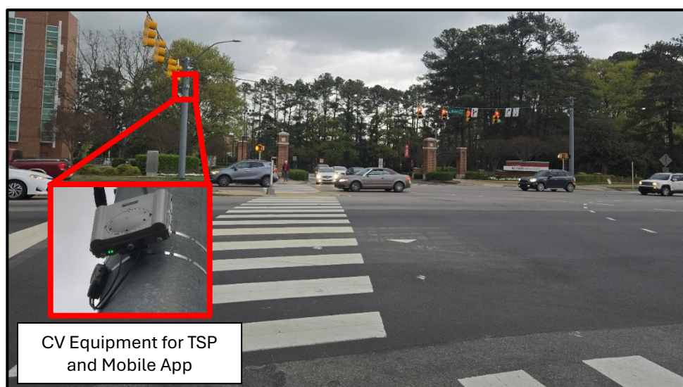
Western Blvd. and Avent Ferry Rd. Traffic Signal and CV Equipment for TSP Operations and Mobile Application for Pedestrians/Motorists
