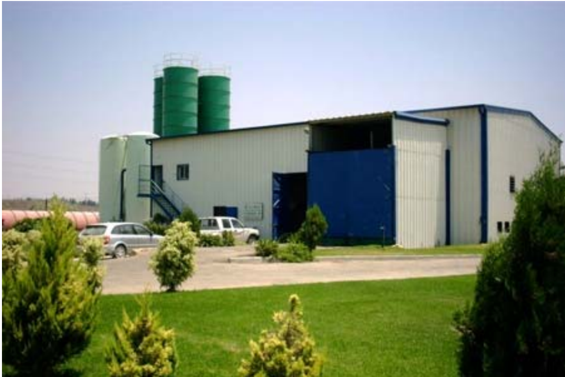
Figure B-14. ArrowBio Facility in Haifa
